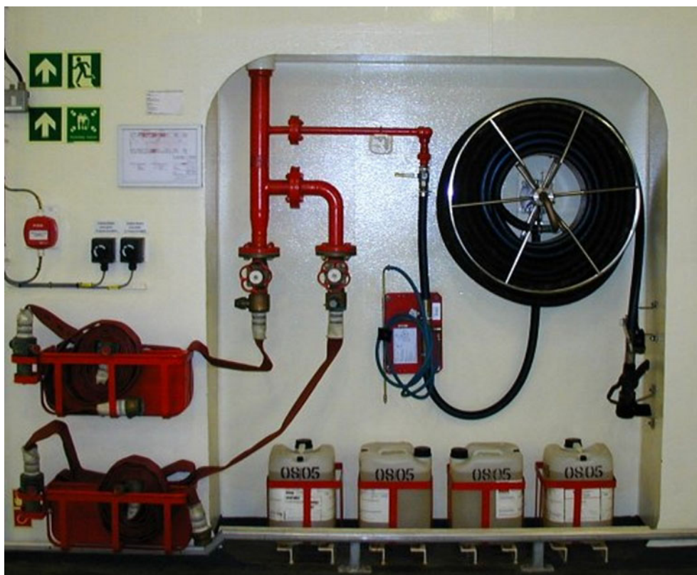
Fig 22-14. Centre Feed (Foam/Water) Hose Reel Unit (Mk 2)
