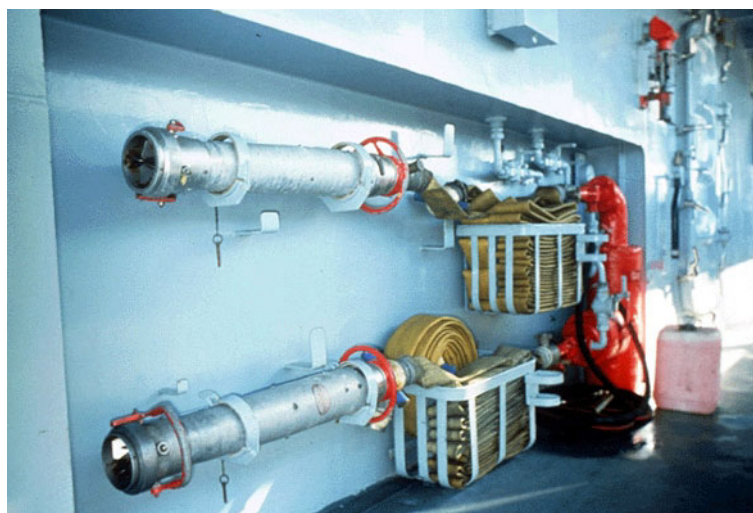
Fig 22-9. Foam Branchpipe FB10(X) or FB10/10
