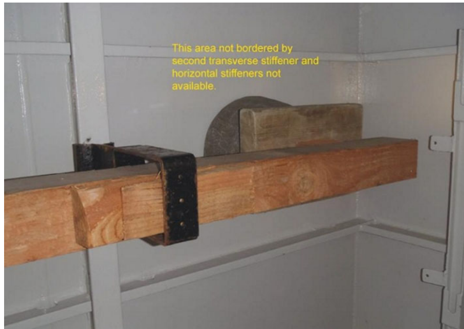
Fig 16-25b. EMMS Clamp Shoring Methods
