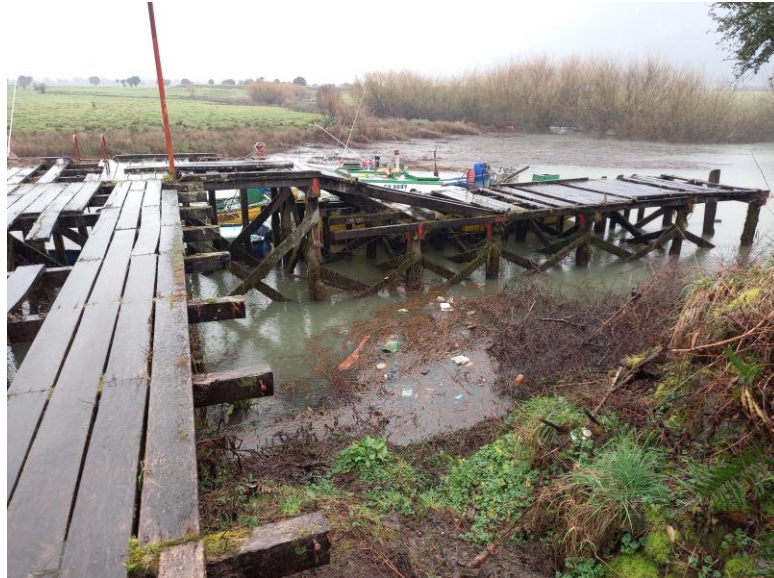
Muelle hospital – Puerto Aysén.
