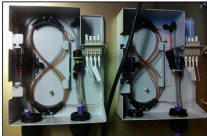
Fig 38H-3. Fibre Optic Patch Panels (FOPP)
