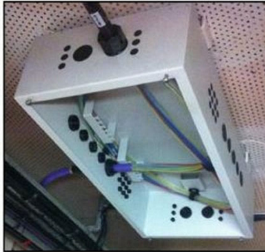
Fig 38H-3. Fibre Optic Patch Panels (FOPP)
