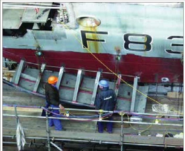
Figure 6: Transom Flap being fitted to a Type 23 frigate
